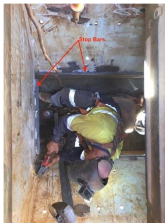
Photo 5 Stop Bars in Place
