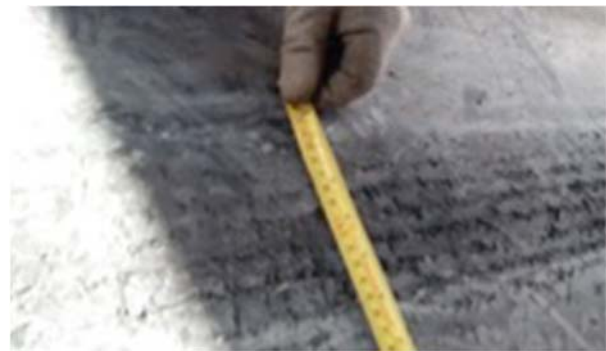
Figure 2 Belt Cover Wear
