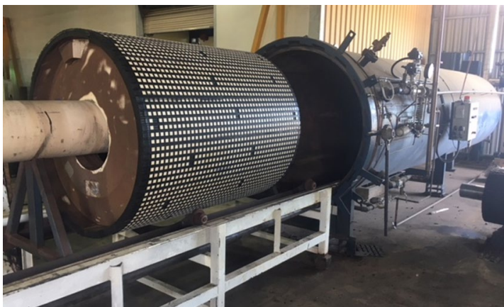
A pulley with Elastotec HVCL being removed from the autoclave
