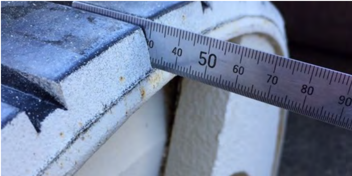
Photo #18. Cold vulcanised lagging gap between lagging strips.
