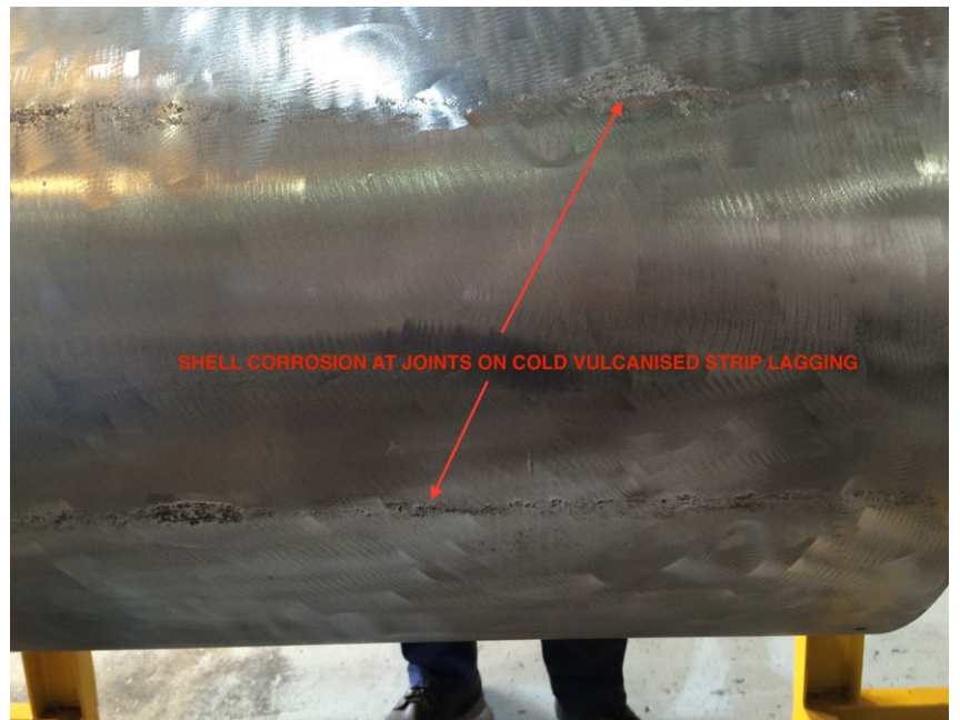
Photo #20. Pulley shell pitting from corrosion due to water ingress between lagging strips.
