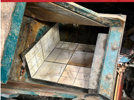
Figure 4. Magnefast™ ceramic wear liners installed on the CG12 chute floor and side wall.
